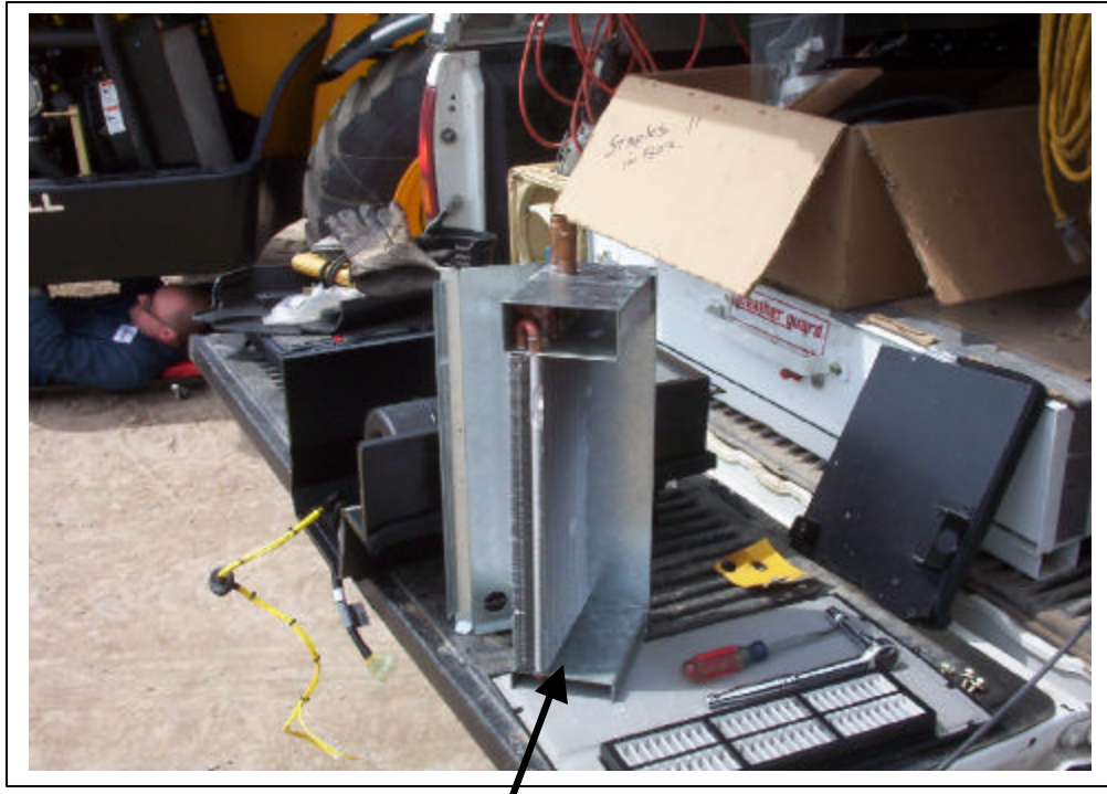
Cut flanges off heater coil flush with heater coil fins.
